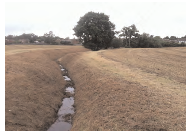
Figure 4.4 Drainage Ditch looking North
