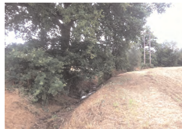
Figure 4.5 Drainage Ditch looking North
